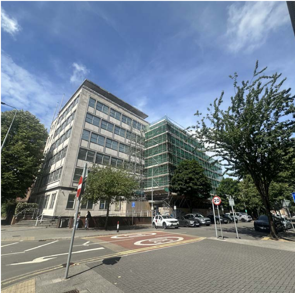
1. South East view of existing building
