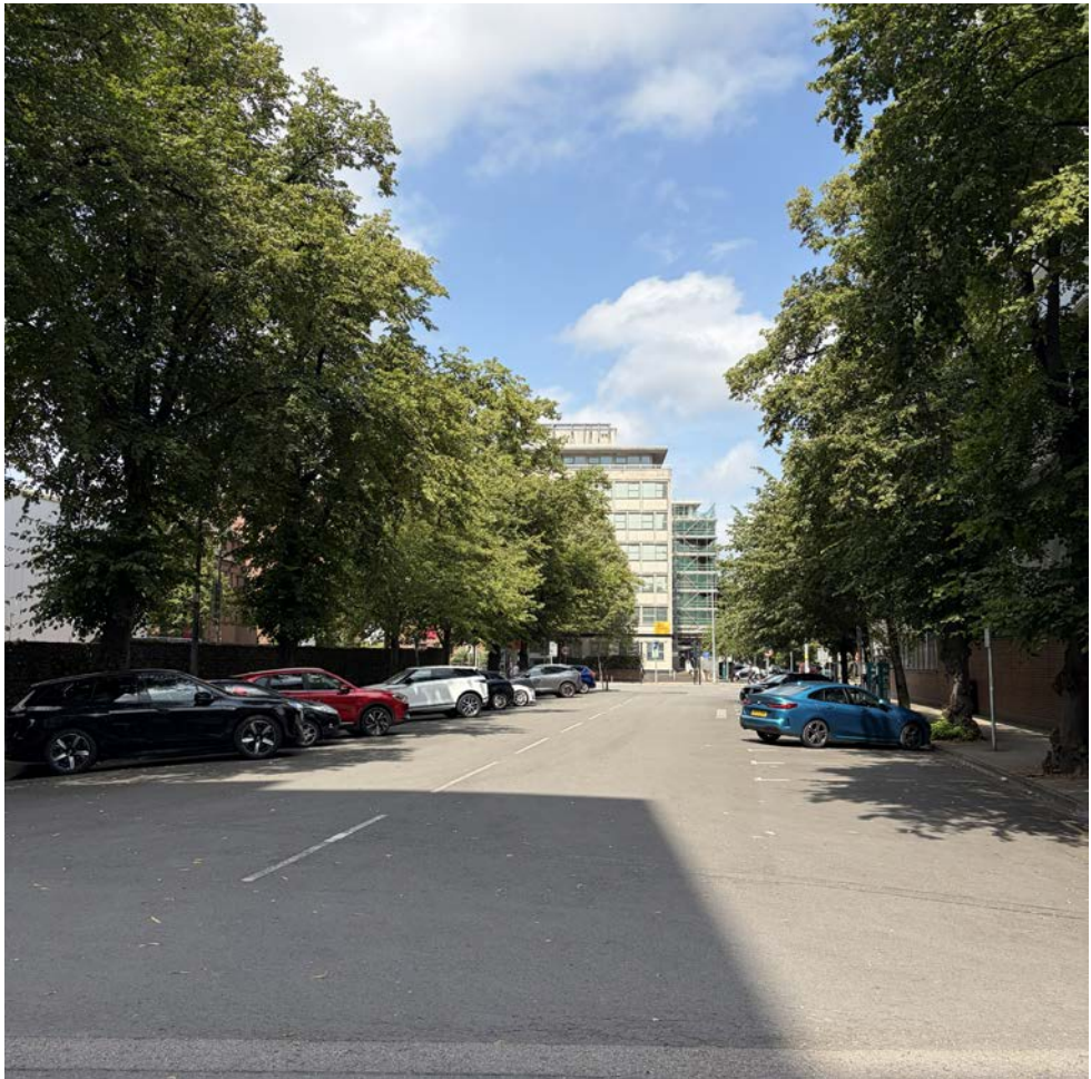
3. South view of existing building from Howard Place
