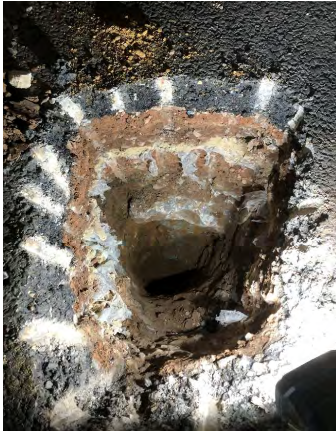
Photograph 7: View of corner of pad foundation encountered within FP01 at ~0.58mbgl.
