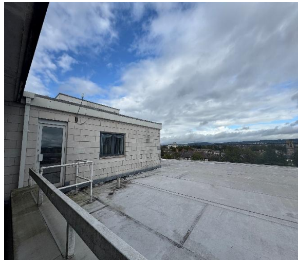
Figure 11 - View of roof.
