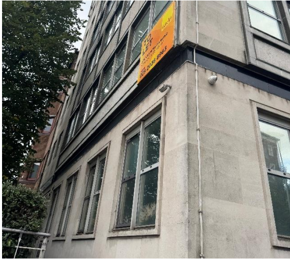
Figure 8 - View of southern side.
