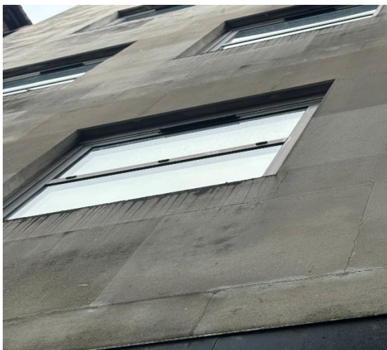
Figure 4 – Example of exterior walls and windows.
