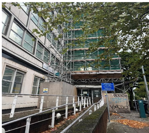
Figure 3 – Scaffolding present on eastern side.
