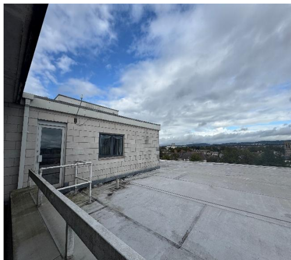
Figure 5 – View of roof.
